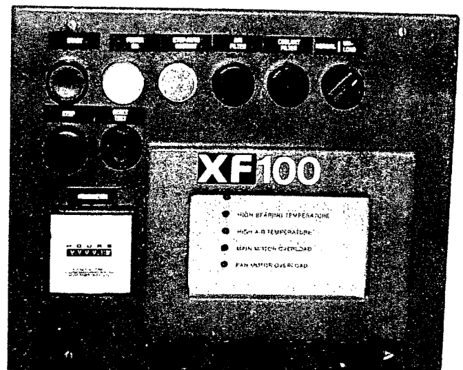
Figure 17A Nema 4/12 Instrument Panel
