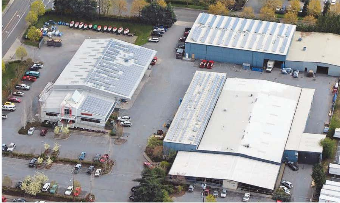
Portland Branch and Corporate Office - Portland, Oregon Offices and manufacturing powered in part by the sun.
