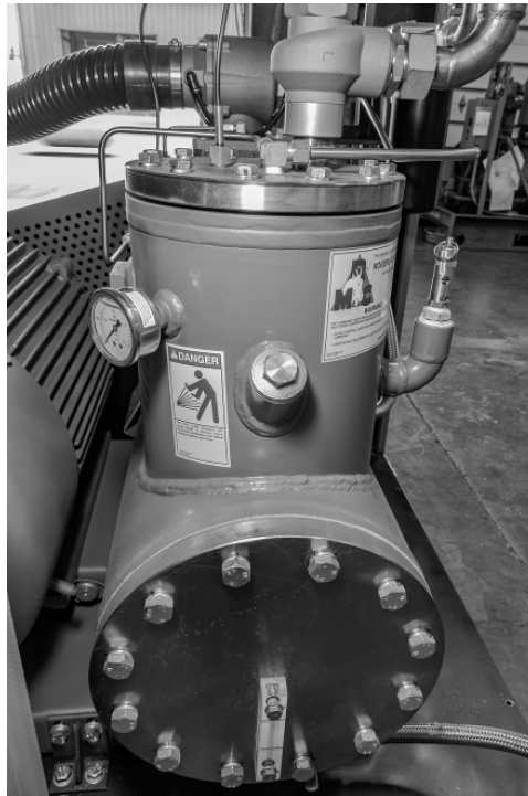
Figure 3. KI Top Hat Style Separator / Reservoir.
